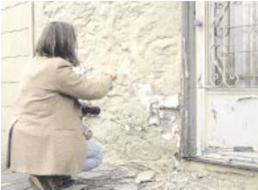
Architectural historian, Kathi Auerbach, points out evidence that the house probably had courting benches flanking the door on the north side of the stone.
