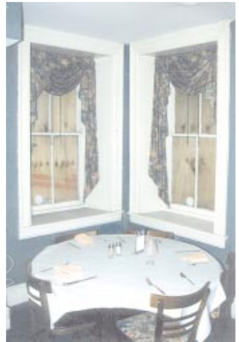
The Tables are still set for dinner! View showing the woodwork details of the Northeast windows of the first floor.
