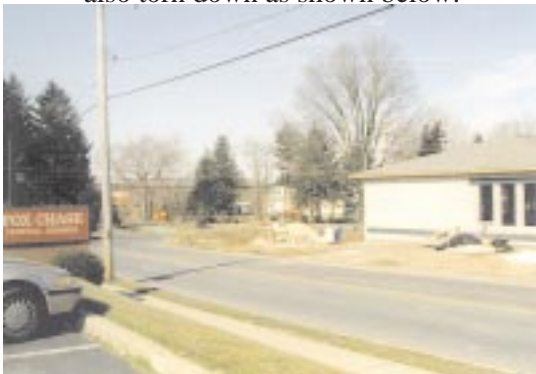
The Victorian house in the background was also torn down as shown below.
