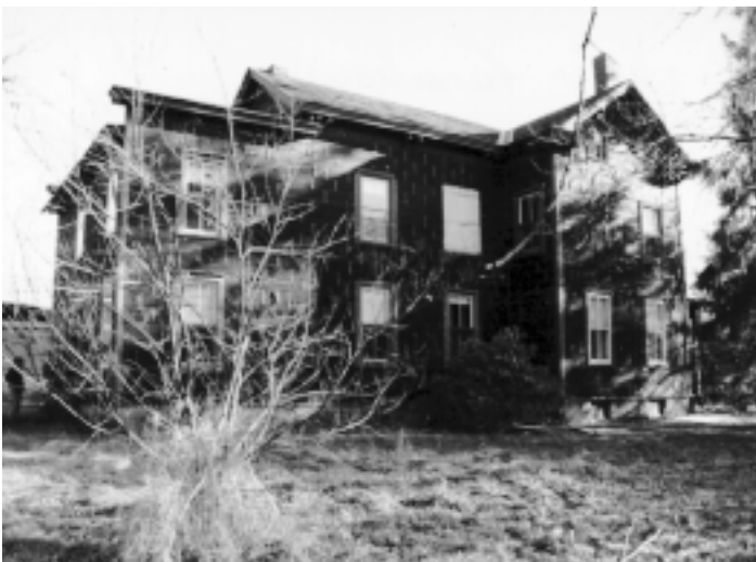
Weir Farmhouse, looking Southeast, Just before demolition. The asbestos siding was removed exposing tar paper over original clapboard siding
