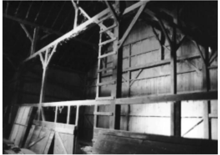
The real beauty of the barn is in it's interior. Classic post and beam construction. One of the finest standing barns in the Richboro area.
