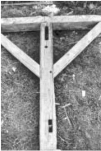
**A reassembled post and beam section. Notice the roman numeral "key" markings**
